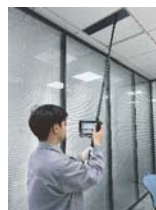
ceiling duct inspection
